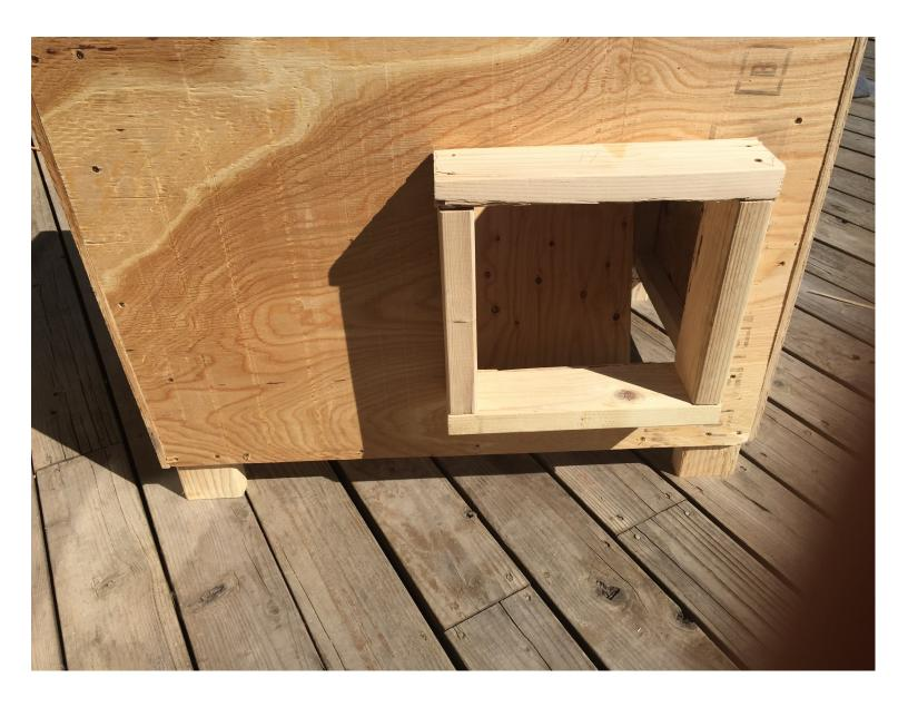
Screw the 19" and the 27" 2x2's around the base to support the loose floor board. (You have to cut corner notches in the floor board so it fits inside the house, which will become obvious).
